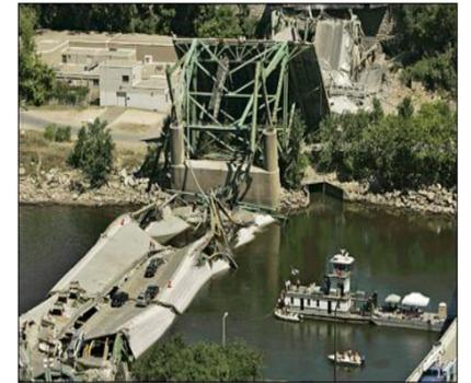
Figure 5 : Collapsed I-35 bridge over the Mississippi river in Minnesota
